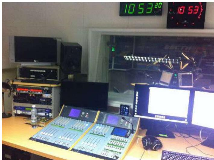
In 2014, the client acquired a redundant Intercom Conexia system for coordination between the studies and technical areas of the radio in Moscow. The installation has 51 user panels for TP4016 rack, one TP5024, 20 TP4216 desktop, and two linkers.
