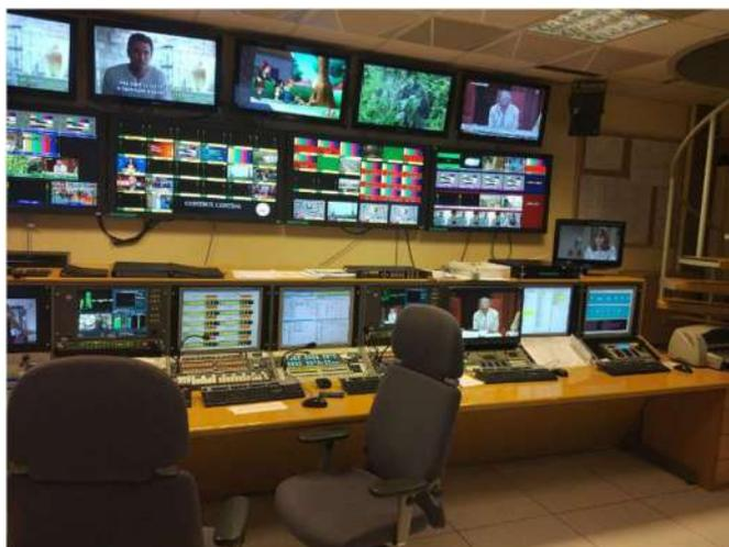
Thanks to the great flexibility of CONEXIA, the project implies a wide variety of panels in order to adjust to TV3's specific needs. TV3 system has 24 and 16-key user panels, with analogue, digital and even AoIP Dante audio.
