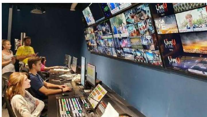
The seven units of TP8000 user panels installed are linked to the AEQ CrossNET matrix, with high quality of audio. In addition to the physical panels, the TV station has added virtual panel licenses to have more workstations.
