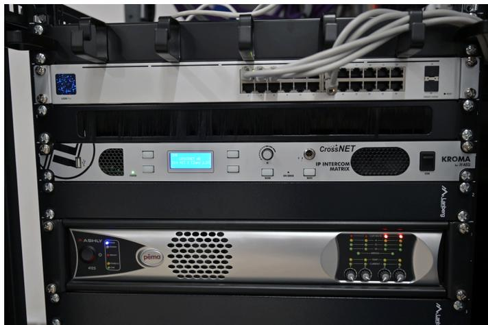
The heart of the system is the intercom matrix CrossNET 40, which is responsible for the audio signal distribution between the rack-mounted TP8116 and desktop user panels TP8416, as well as the Wi-Fi based wireless belt packs AEQ XPLORER and can be used not only for audience paging but also to broadcast for example, narration or voice over.
